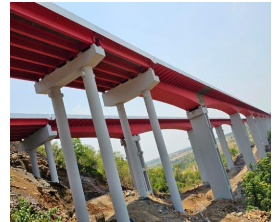
SAMRUDDHI MAHAMARG (AFCONS INFRA) (Fly Over Civil Structure)
