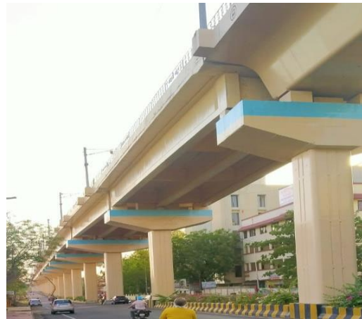
NAGPUR METRO IPN TECHNOLOGY PAINT SCHEME (Metro Civil Structure)
